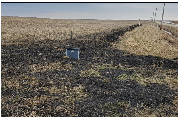
Saturated buffer recently installed. Photo by Emery Davis.
